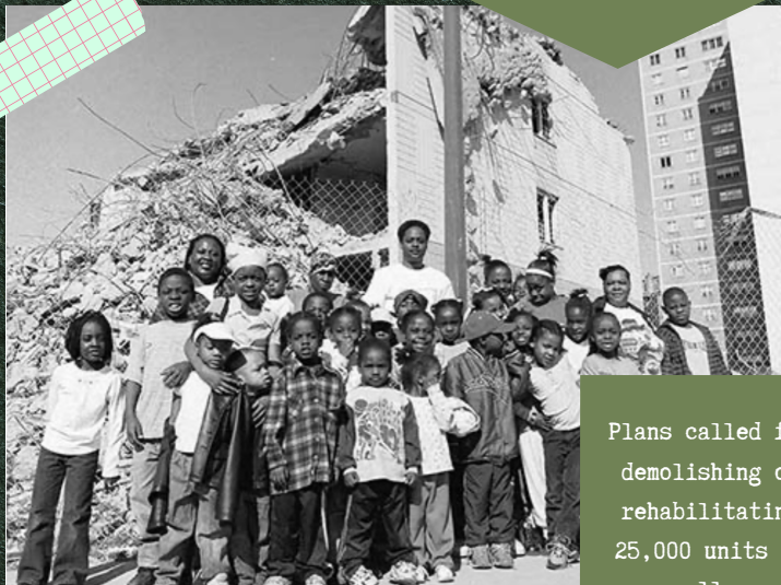
Former Stateway Gardens residents standing in front of demolished building, 2001
