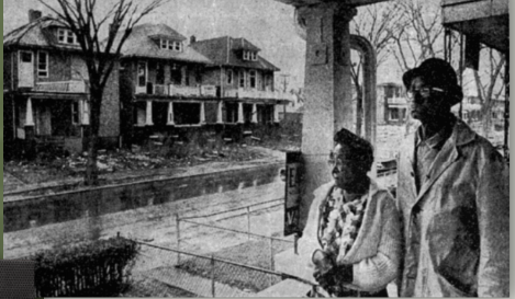
James and Katie Nicolson standing on their porch looking at destroyed homes, 1973
