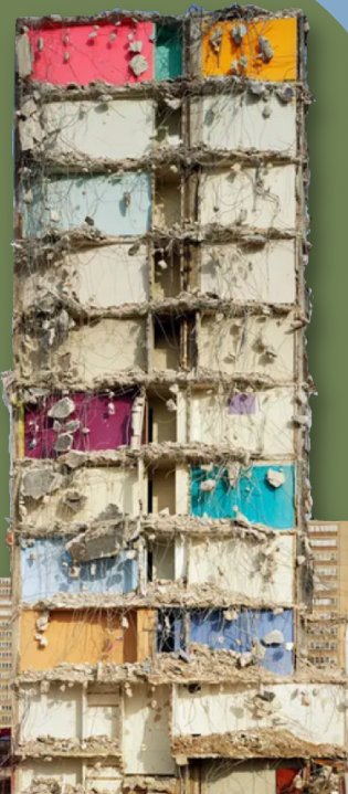
Partly demolished Cabrini-Green building, 2006
